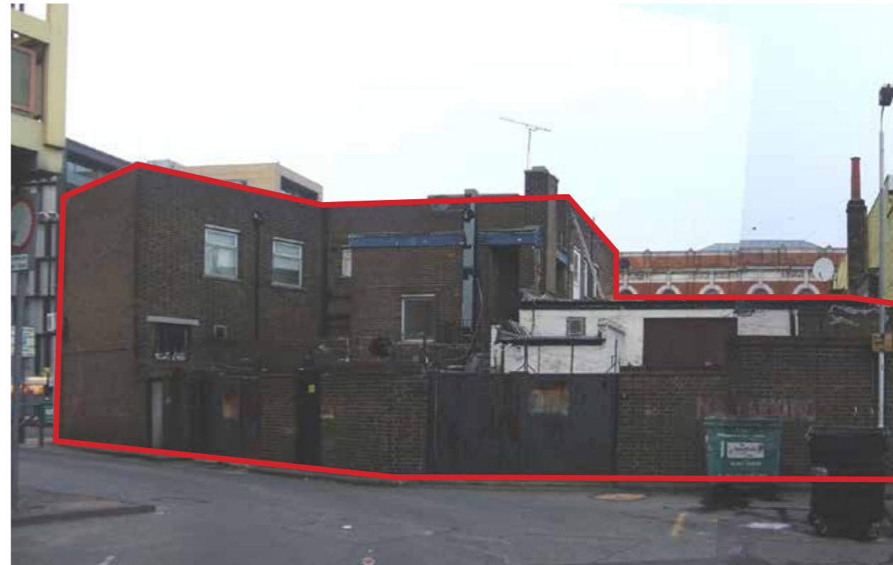
2. View of the rear of the existing site
